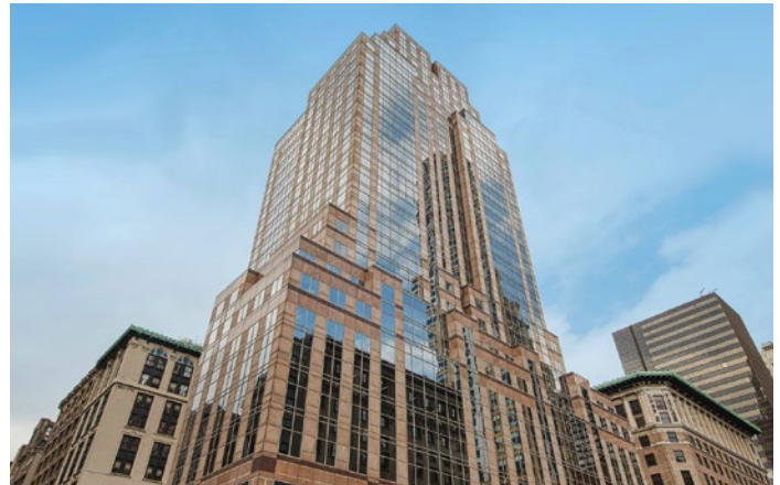
The distressed developers of 420 Fifth Avenue turned to an office condominium conversion strategy to save their buildings and turn a profit
